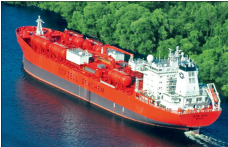
Fig. 6.23. A chemical tanker of B 588 series with tanks seated on the deck by using EPY compound EPY
