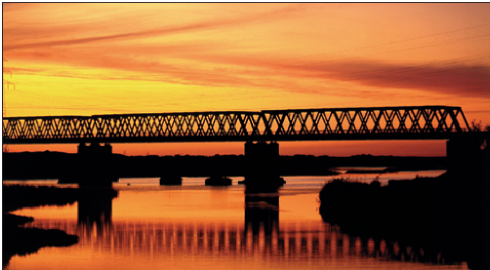
Fig. 6.67. Railway bridge in Wolin with bearings seated (in 1994) on EPY compound chocks (acc. the scheme shown in Fig. 6.66a)
