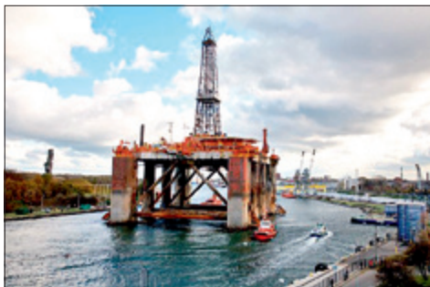
Fig. 6.33. MODU "Bredford Dolphin"; main propeller electric motor was seated under supervision of DNV; the work was performed in Gdansk Ship Repair Yard (2007)
