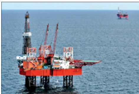
Fig. 6.32. MODU "Petrobaltic" and "Balic Beta"; on the first drilling unit a windlass (in 1984) and electric generator (in 1994) was seated; the operations were performed in the Ship Repair Yard "Radunia"; on the second unit three WAB 1240 D6 electric generating sets and three supporting bearings were seated; the operations were performed in sea conditions (2004÷2005)
