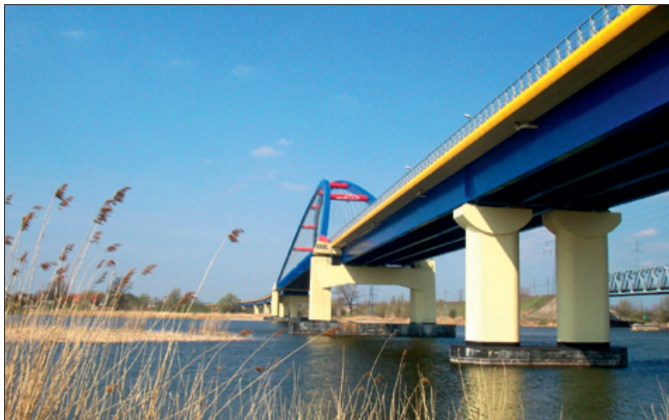
Fig. 6.69. A bridge and a trestle bridge along the train of Wolin ring road, with bearings seated by using EPY compound
