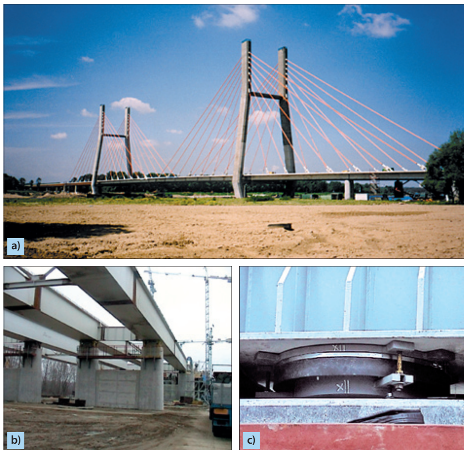
Fig. 6.68. The “Siekierkowski” bridge under erection in Warsaw (2001): a) overall view; b) view of bridge span; c) view of a span bearing seated by using EPY compound (acc. the scheme shown in Fig. 6.66d)
